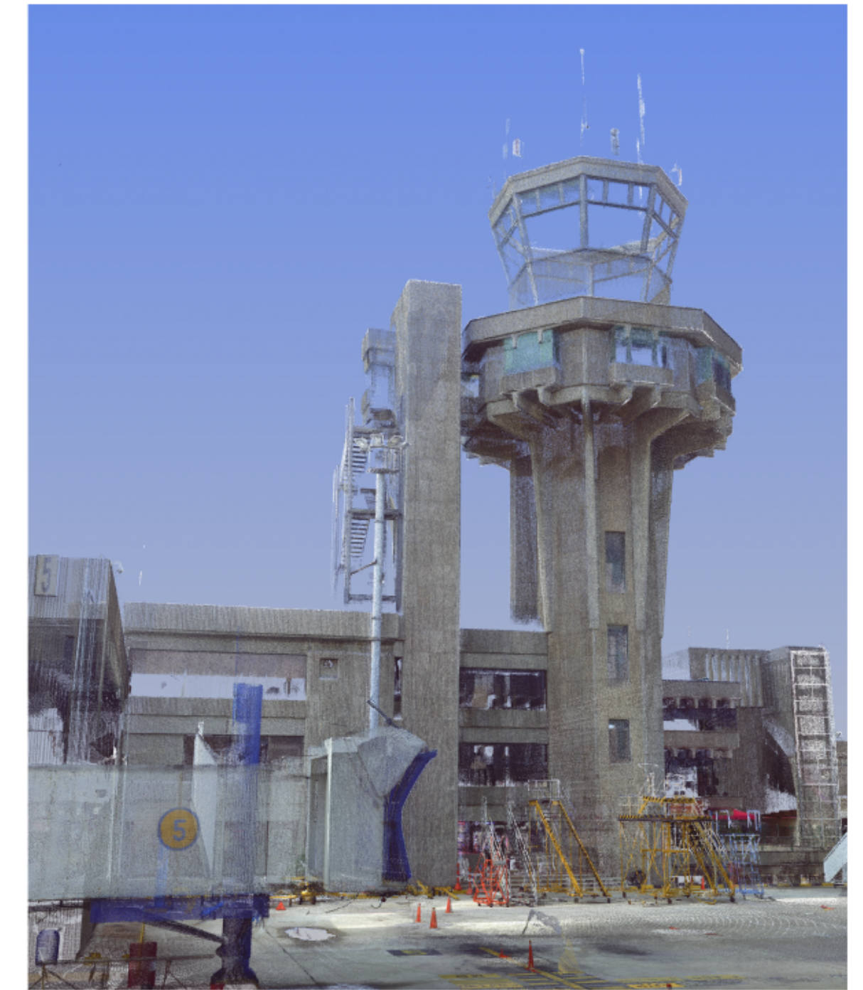
perspective view of the BAQ airport in Colombia - point cloud only
